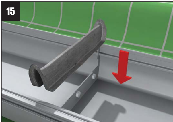
Dress the joint with lead.
