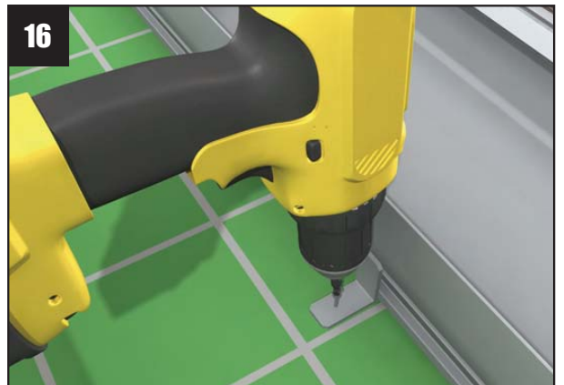
Screw fix the box gutter down to the structural cassette using the brackets supplied.
