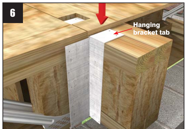
From the top, tap down the hanging bracket tab and secure in place using 65mm round head nails.
