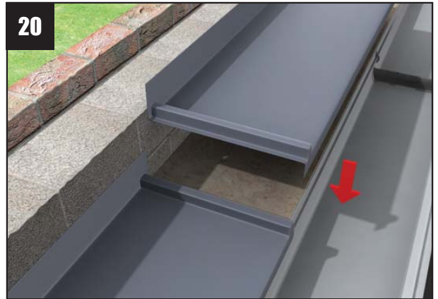
Having raised the masonry to its finished levels, lay the pre-formed GRP panels into position.
